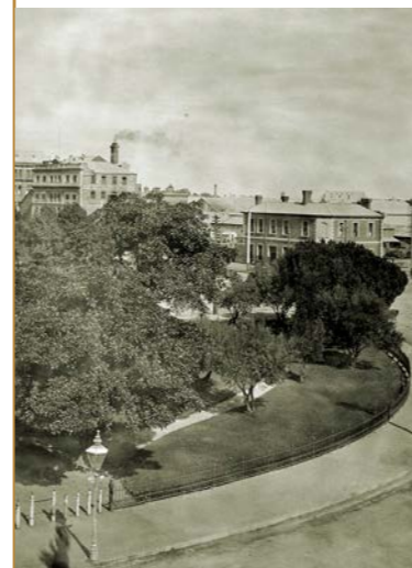
A 1911 photograph taken from the northern portion of Light Square.
